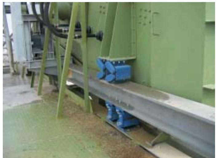
Fig. 2: Gravel dewatering screen with counter-frame on ROSTA AB's and AB-D's
